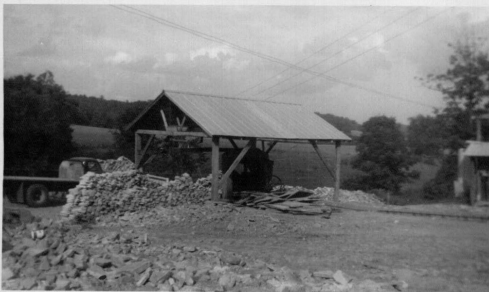
Figure 64. A wire saw for cutting stone.
