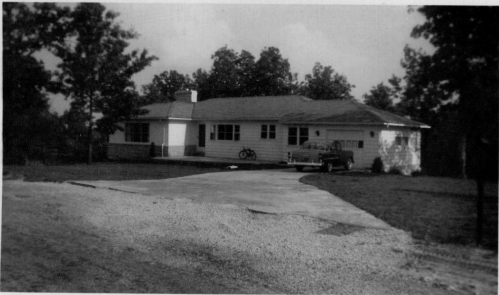
Figure 14. A typical home in Volunteer Heights, a modern subdivision south of the Crossville city limits.
