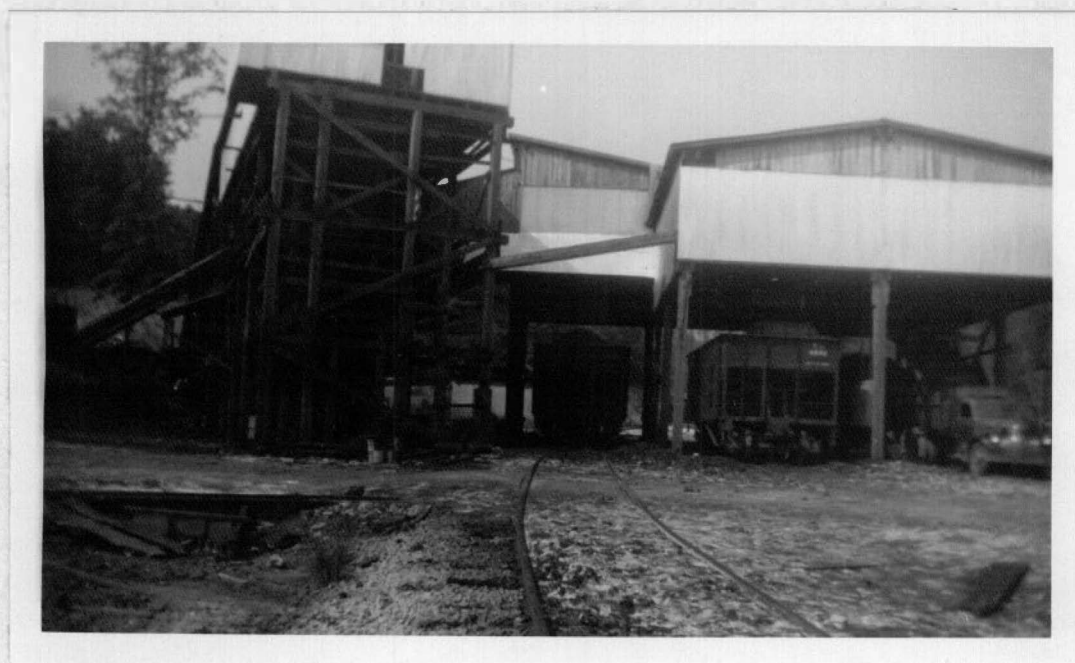
Figure 54. The coal loading tippie for the mine at Isoline.
