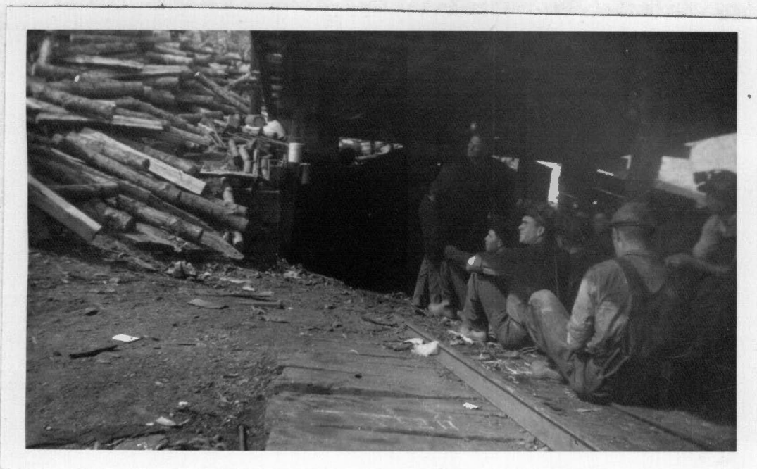
Figure 53. The entrance to the "slope" mine at Isoline in the northern part of Cumberland County.
