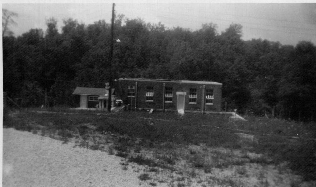
Figure 72. The filtration plant of the Crossville municipal water system.
