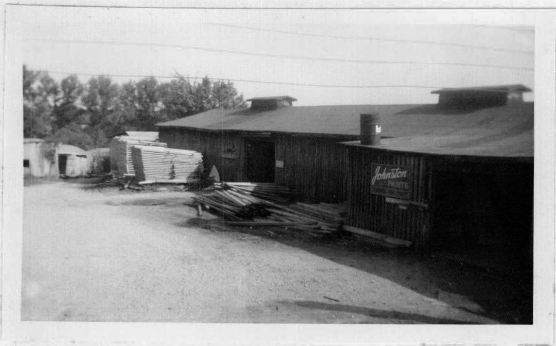
Figure 82. The C. R. Graybeal and Sons house construction materials plant.
