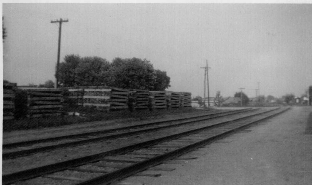
Figure 74. The crosstie concentration yard and Tennessee Central Railroad siding at Mayland.
