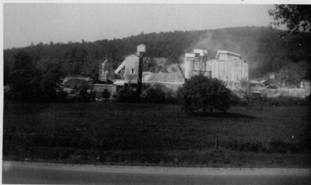
Figure 69. Limestone crushing mill of the Southern States Lime Corporation works at Crab Orchard.
