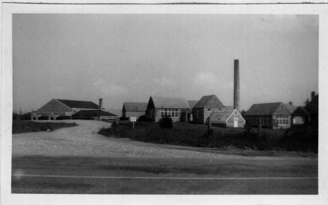
Figure 24. The Cumberland Homesteads community center.
